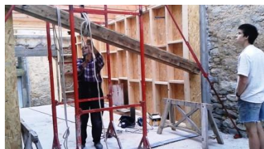
Oak beam installation with Grégoire
