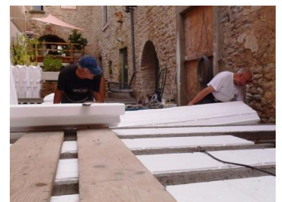
Making the insulating floor with Alfonso
